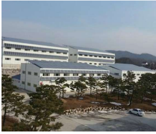
SH Logistics Center (1,500 kW)
