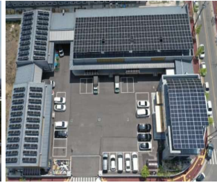
Ulsan Ulju Factory Rooftop (200 kW)
