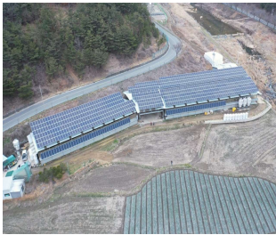
Sancheong Livestock Facility Rooftop (350 kW)
