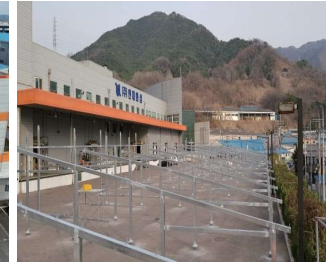
Industrial Complex Rooftop and Parking Structure (1,000 kW)
