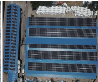
Sancheong Livestock Facility Rooftop (300 kW)
