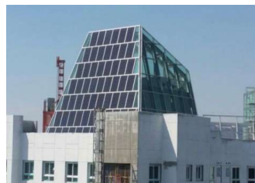
Masan Metro City – 53rd floor rooftop installation
