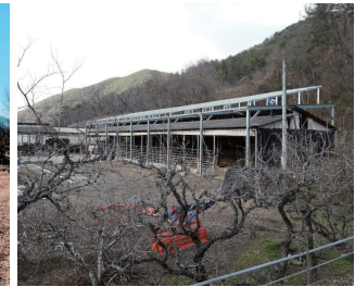
Miryang Livestock Facility – Reinforced Slate Roof (100 kW)
