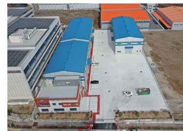
Ulju-gun Factory Rooftop – Phase 2 Project (500 kW)
